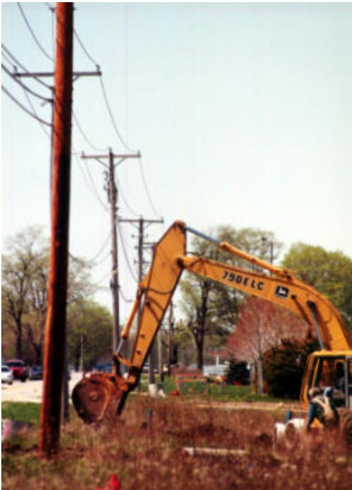
***Excavators & backhoes*** are similar to drilling rigs in that they too require consideration both overhead and underground. Many types of work that requires the use of excavating equipment often take place along side of roads where power lines are present. By utilizing equipment with limited reach potential and not storing pipe, trench boxes and other material underneath power lines can reduce the likelihood of a contact.
