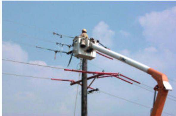
If insulated sleeves are used, power company personnel can only install them and they must be appropriate for the type of work being performed. Workers have been electrocuted when insulating sleeves have failed and the equipment they were working with became electrified. So, never work closer than the line clearance distance.
