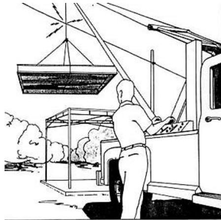
Workers installing a chain link fence directly under an overhead power line were electrocuted when one of the workers raised a long section of top rail and brought it into contact with the line.
